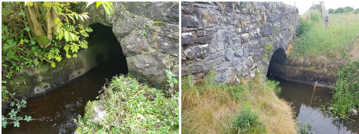
Plate 2 Underpinned road culverts along the Drum tributary Stream
